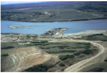
Lake Diefenbaker Construction in the 1960s
